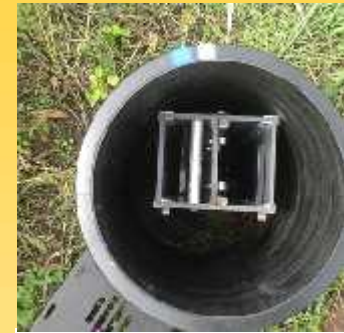
Control drainage structure
